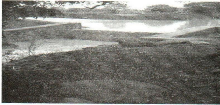
Figure 6. Low-cost Water Harvesting Structures in Wadgaon Village of Yavatmal District
